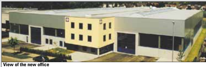
View of the new office
