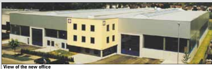
View of the new office
